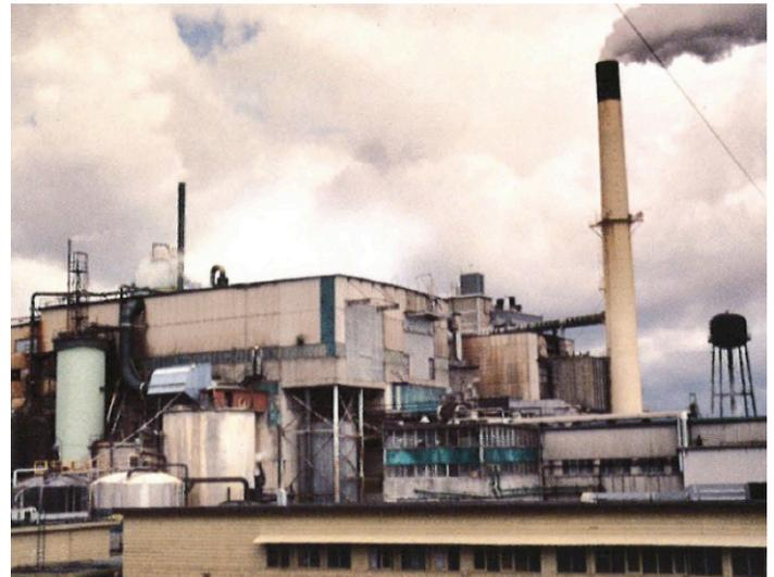
The composition of the flue gasses is typical for a kraft pulp mill and includes carbon dioxide, oxygen, sulfur dioxide, reduced sulfur, water and particulates.
